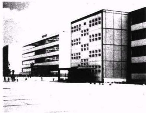
Identical construction reduces costs of new Ten-Year Schools.
