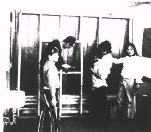
Websterville businesses are constructed with wooden frames covered by paneling.
